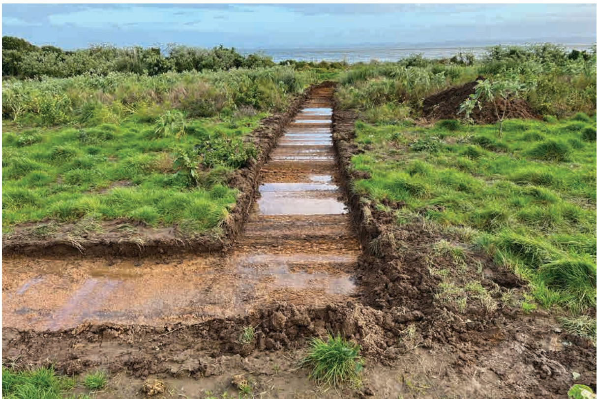
Figure 6. Trench 4, with water seeping in.
